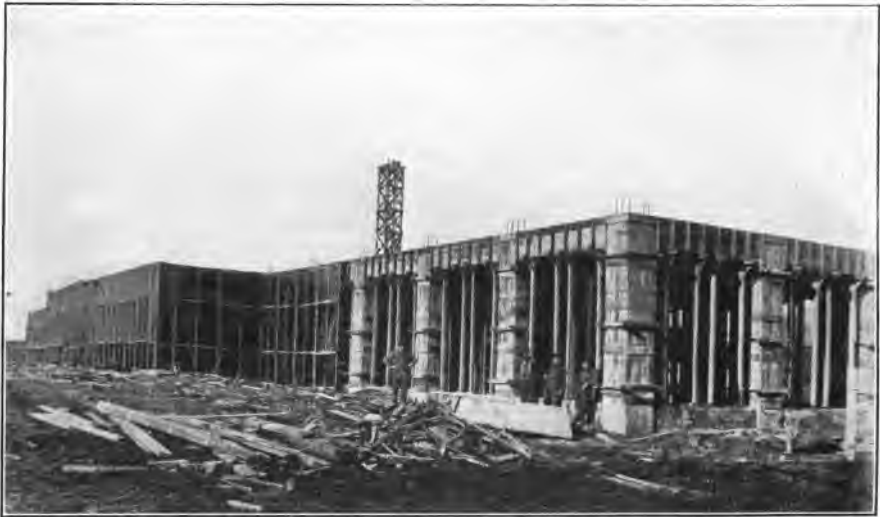
FIG. 12.—USE OF PAPER-COVERED FRAMES FOR ENCLOSING BUILDING.
